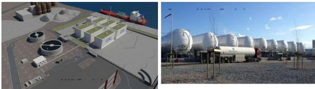
Figure 117: Exemples de terminal PTS de type mid-size bullet cylinders
