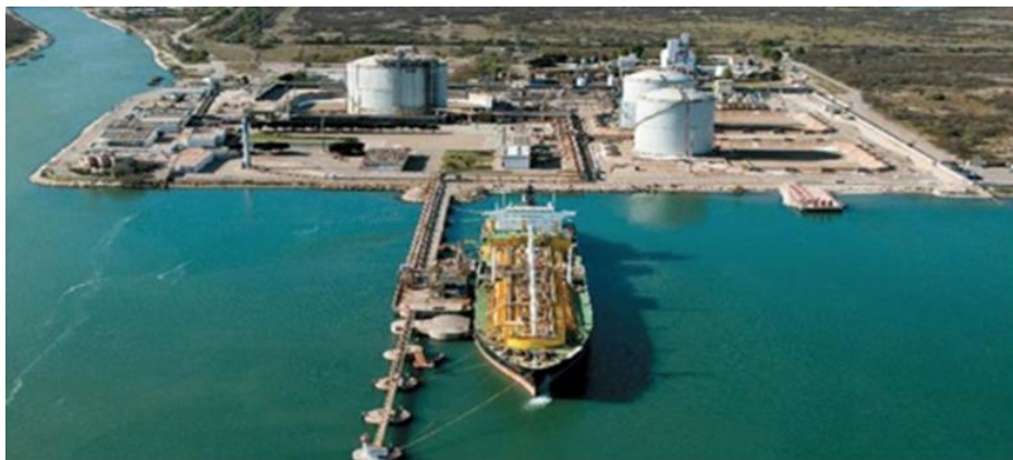
Figure 31. Terminal GNL de Fos Tonkin
